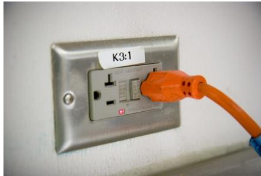
Figure 8-3: 3-Prong Outlet with GFCI
