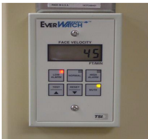
Figure 6-9: Through-the-Wall Velocity Sensor
