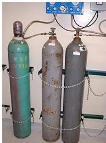
Figure 8-7: Proper Cylinder Restraint (In a seismic area, two chains are required.) (Source: University of California, San Diego , 2011)
